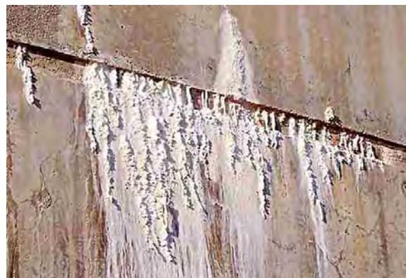
Figure 6 Efflorescence as seen on block faces (b)
